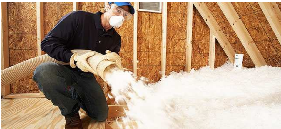
Figure 3: A construction worker spraying loose fill insulation material in the roof of a new construction [20]
